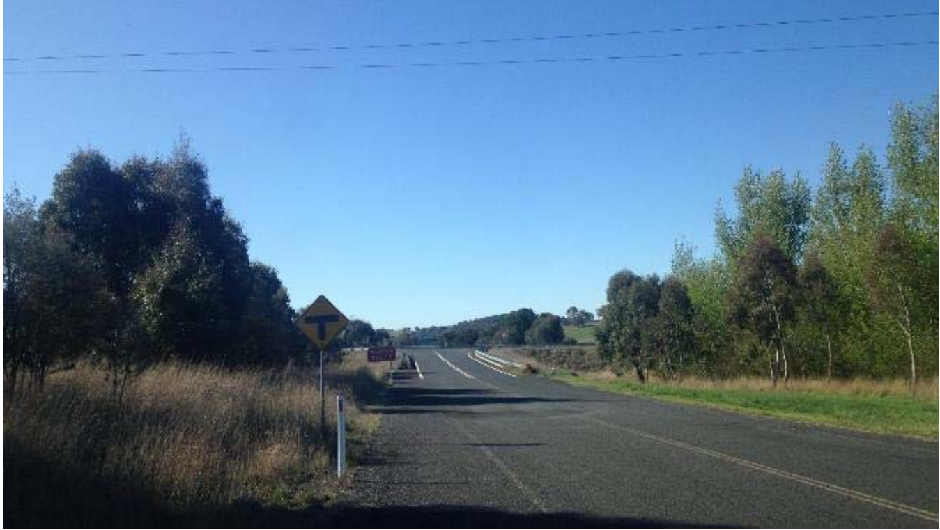
Plate 11: The Great Western Highway/Walkom Road West intersection looking north
