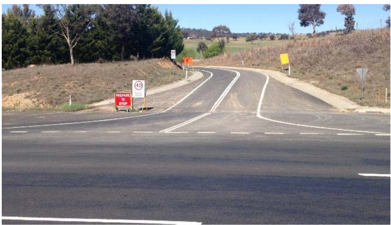
Plate 7: The Great Western Highway/Hen and Chicken Road intersection looking east
