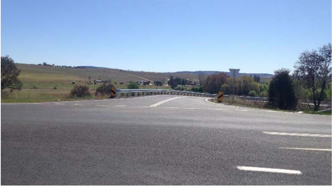
Plate 9: The Great Western Highway/Evans Plain Road intersection looking east
