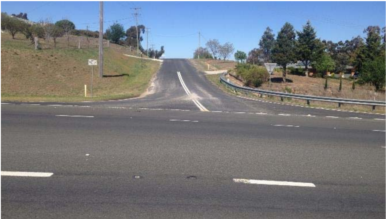
Plate 6: The Great Western Highway/McLennan Close intersection looking south east
