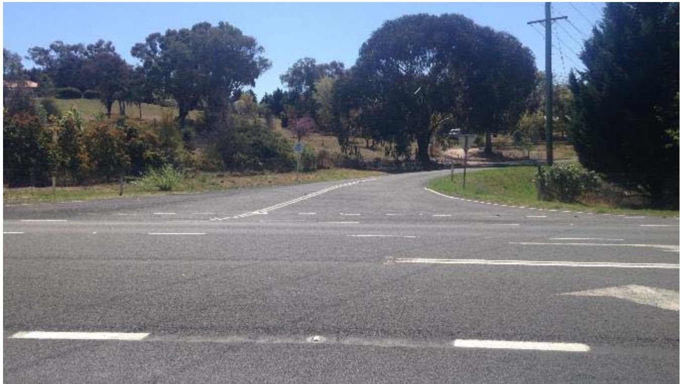
Plate 4: The Great Western Highway/Delaware Crescent intersection looking north
