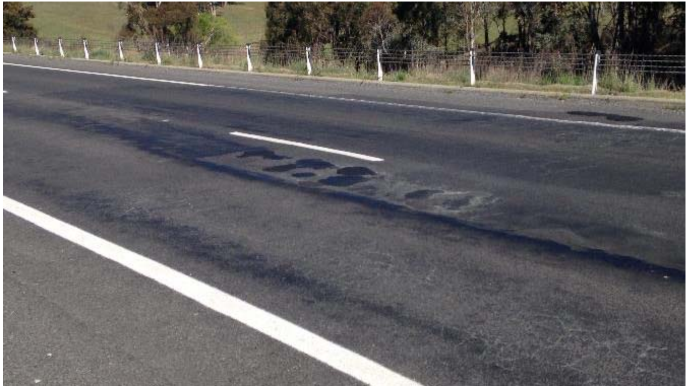
Plate 22: Block cracking, stripping of aggregate, loss of texture and moderate deformation – evidence of repairs
